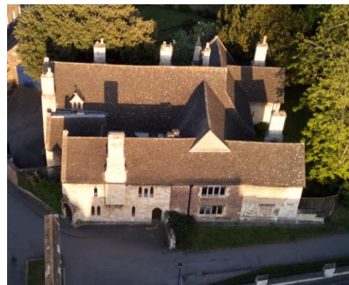
Aerial View of Dulverton House
