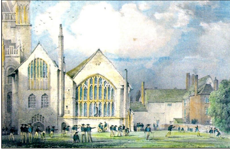
A painting showing the 'Babylon' buildings alongside the Chapter House. This painting is before 1849, when the schoolroom was built.
