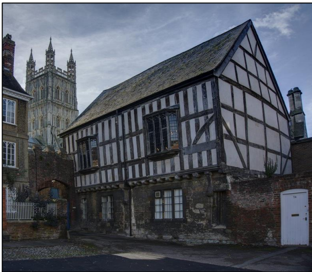
The timbered framed room sitting on top of the earlier medieval base
