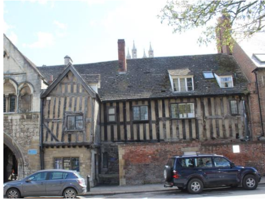
The rear of No 14.
