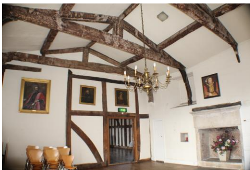
The painted medieval beams in the roof of the Henry Room. The view shows the entrance to the Parliament Room
